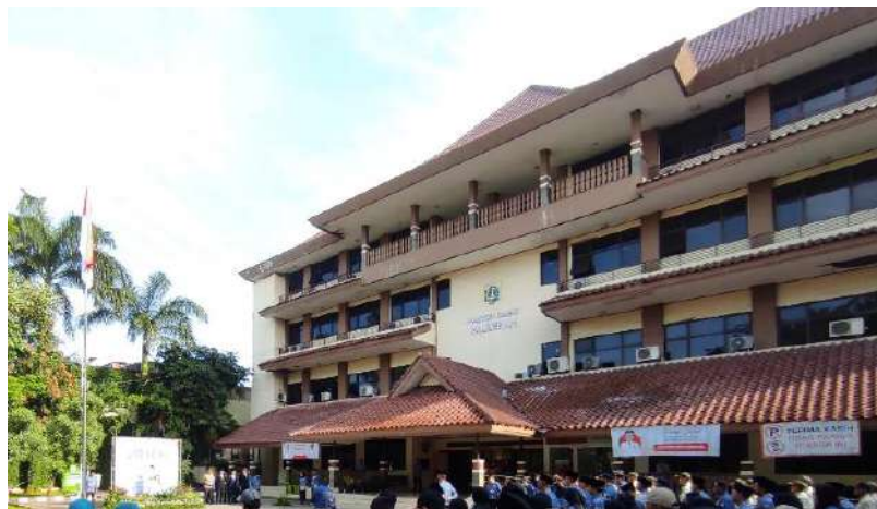
Figure 4. Palmerah District Office Building
