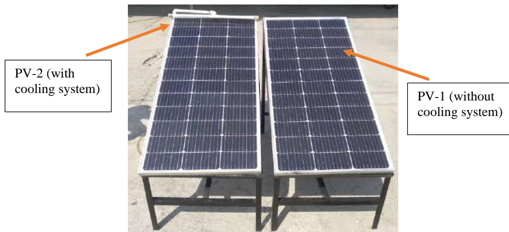
Figure 7. PV panels configuration
