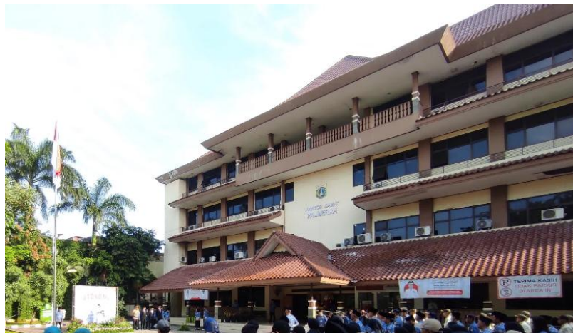
Figure 4. Palmerah District Office Building
