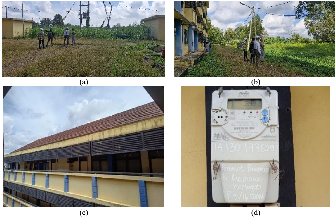
Figure 3. Site visit, (a) and (b) show the placement options for the PV panels in open fields available at the location. (c) Shows the placement options for the PV panels at the rooftop location. (d) A 3-phase meter
